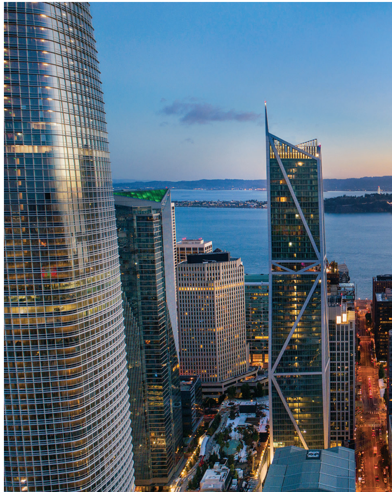
Thermafiber ® FireSpan ® mineral wool insulation provided critical components of the perimeter fire containment system in 181 Fremont in and San Francisco, CA. Photography credit: Jay Paul Co.
