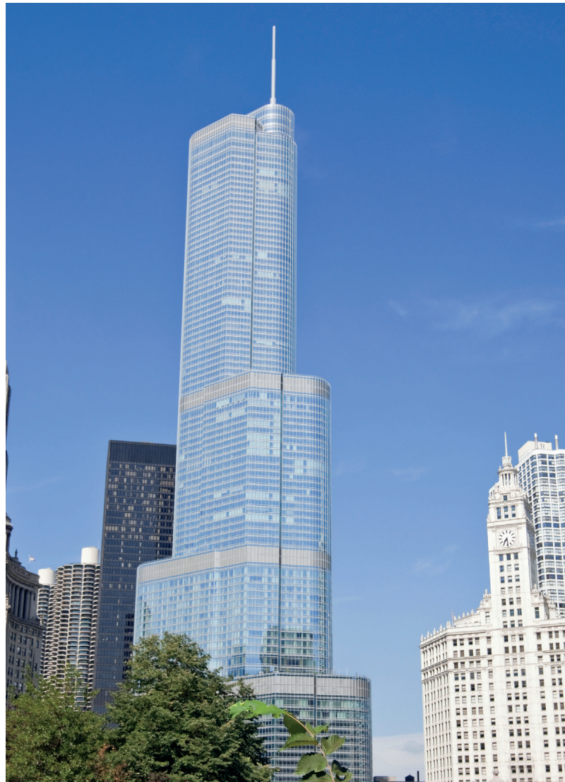
Thermafiber® FireSpan® mineral wool insulation provides the critical components of the perimeter fire containment system in the Trump International Hotel and Tower in Chicago, IL.
