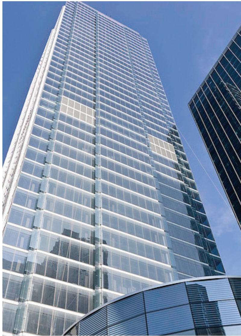
The Thermafiber® Impasse® Insulation Hanger System was used to install various Thermafiber® mineral wool products in the perimeter fire containment system at 353 N. Clark in Chicago, IL. Thermafiber® mineral wool insulation contributed to this building's LEED® Gold status.
